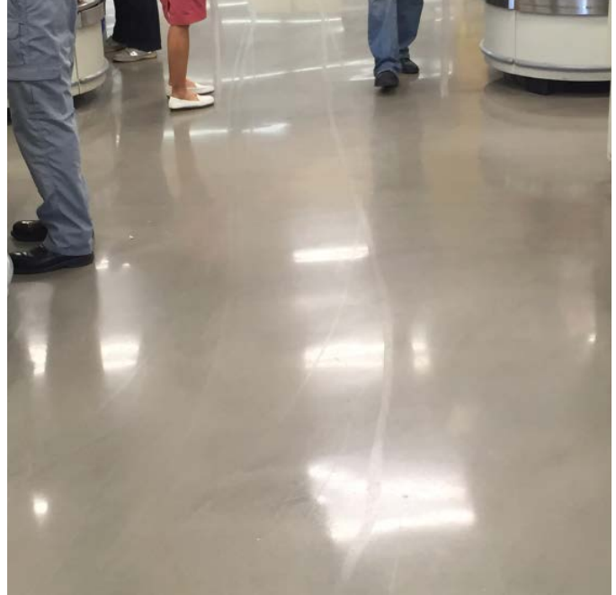
Aggregate in an overlay makes a surface more impact resistant. It helps stop “denting” or impressions from occurring when a heavy weight is rolled across the floor or dropped on it.
