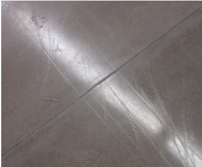
Aggregate in an overlay makes a surface more impact resistant. It helps stop “denting” or impressions from occurring when a heavy weight is rolled across the floor or dropped on it.
